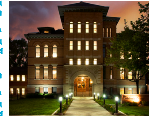
The front façade of the Oquirrh School Building at twilight.
